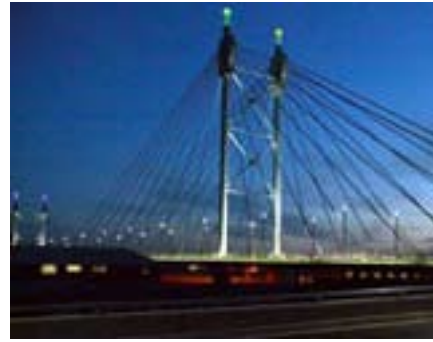
The Nelson Mandela Bridge, Newtown
