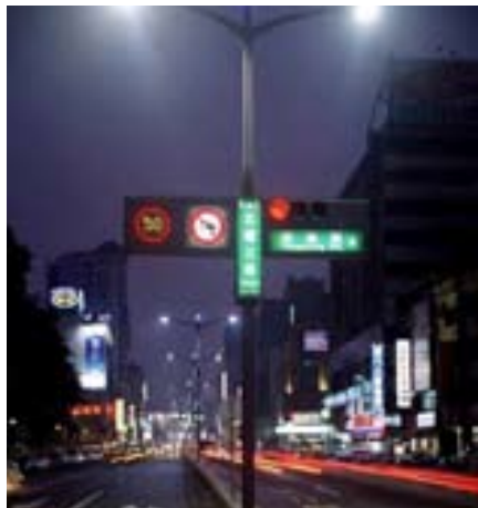
Utilization of solar power in Street Lighting, City of Kaohsiung. (Charles Lin)
